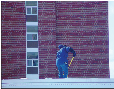
Figure 2.153 Snow removal duties, around and on top of the trailer. Some trailers have heaters where the expandable sides mate with the rest of the trailer. If snow accumulates in that area and freezes retracting the expando might prove difficult.
